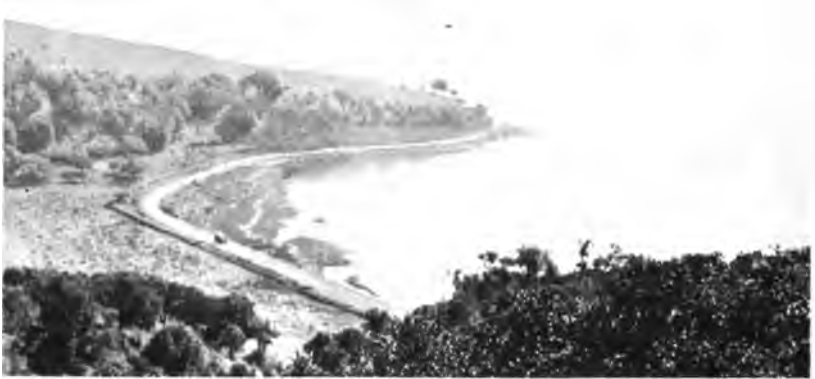
A birdseye view of Bolinas Bay and shore line drive.
